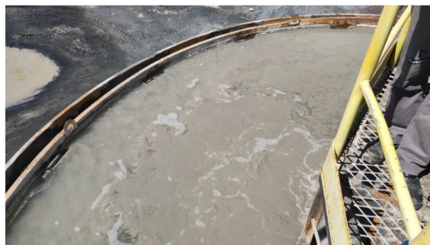
Figure 2. View of one of the chromite tailings thickeners operating at Ipuera/FERBASA.
